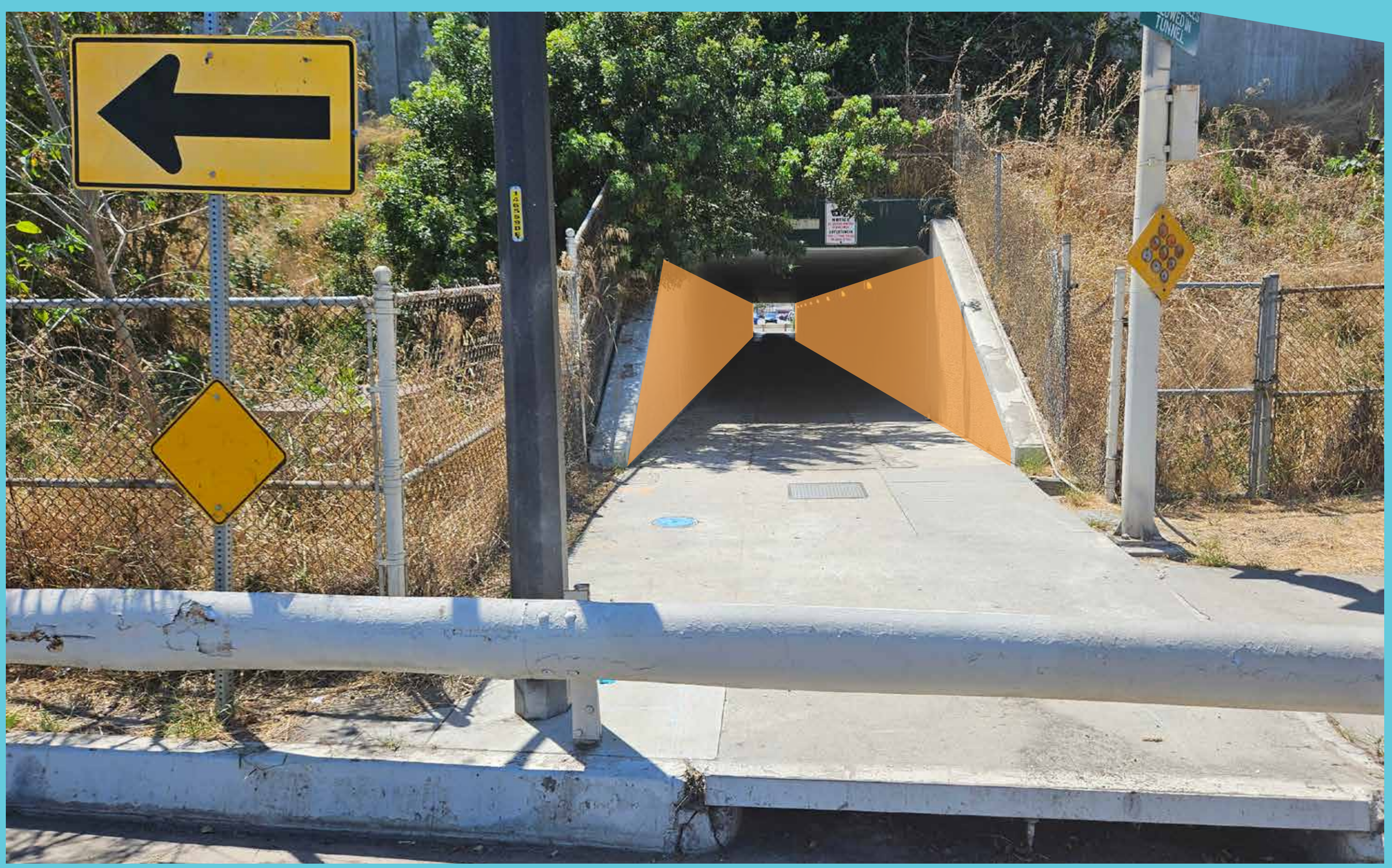
VIEW FROM 710 FREEWAY UNDERPASS AT LEONIS ST
